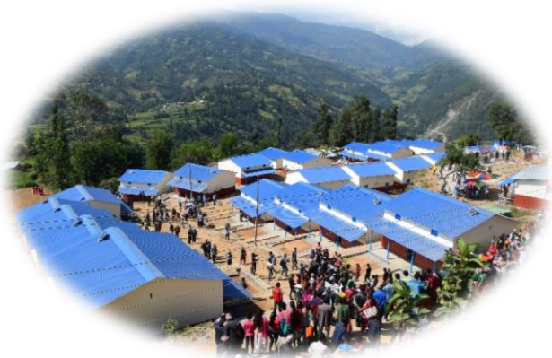
Solar panel support in Giranchaur, Sindhupalchowk
