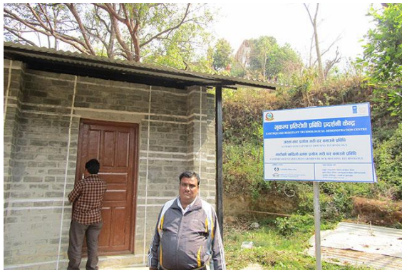
Compressed Stabilized Earthen Block (CSEB) Demonstration House, Saraswati HS School, Gorkha Bazaar, Gorkha
