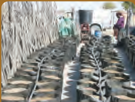
Installing of an irrigation system
