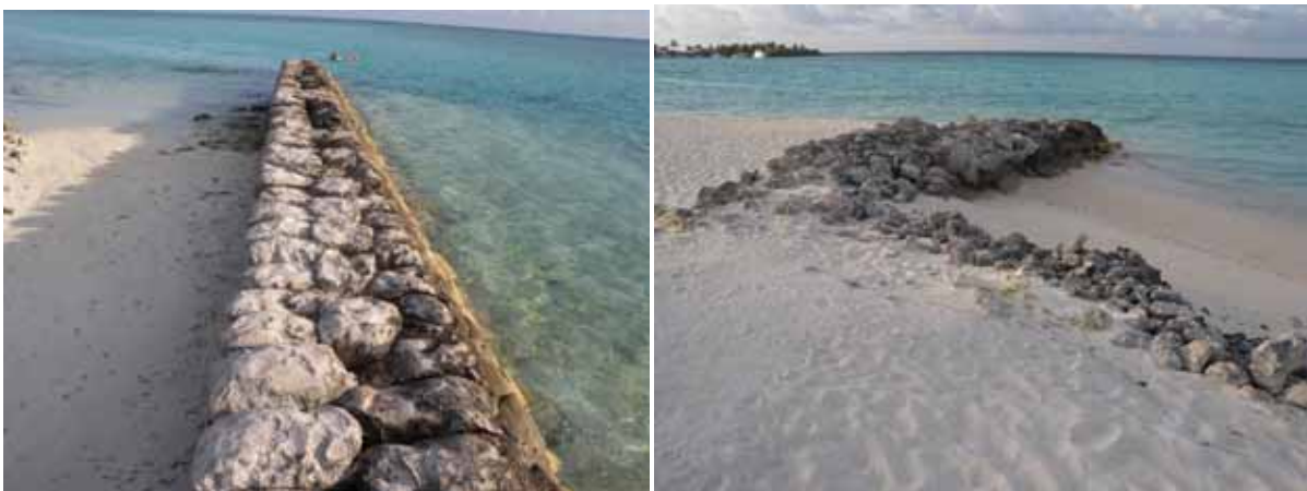
Figure 4.27 Groynes constructed from coral rubble in B. Reethi beach and AA Bodufolhudhoo
