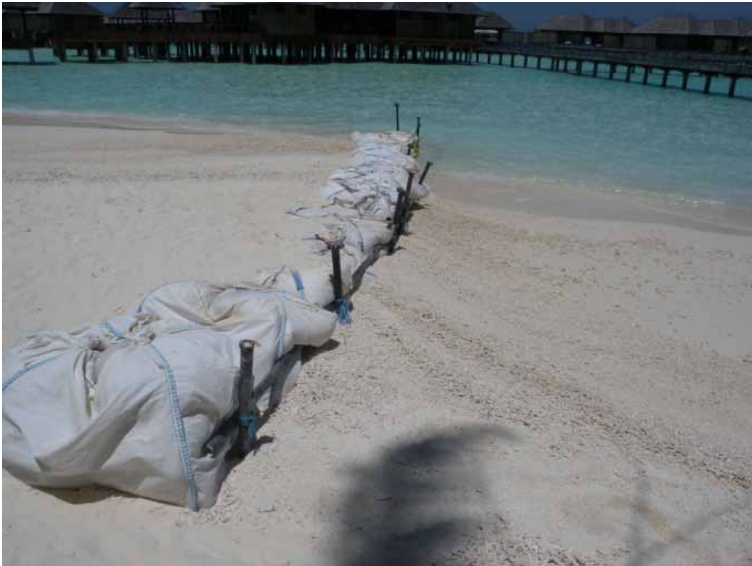
Figure 5.2: Temporary groynes constructed in N. Irufushi Island
