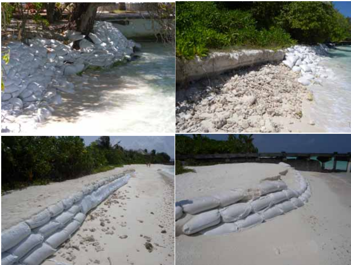
Figure 5.3: Temporary groynes constructed in N. Irufushi Island
