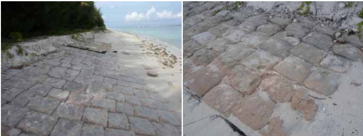
Figure 4.23: Generic revetment design – Rubble slope with concrete plastering in K. Boduhithi
