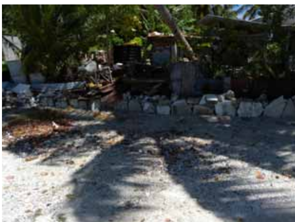
Figure 5.17 Use of both construction debris to protect properties from flooding in S. Feydhoo
