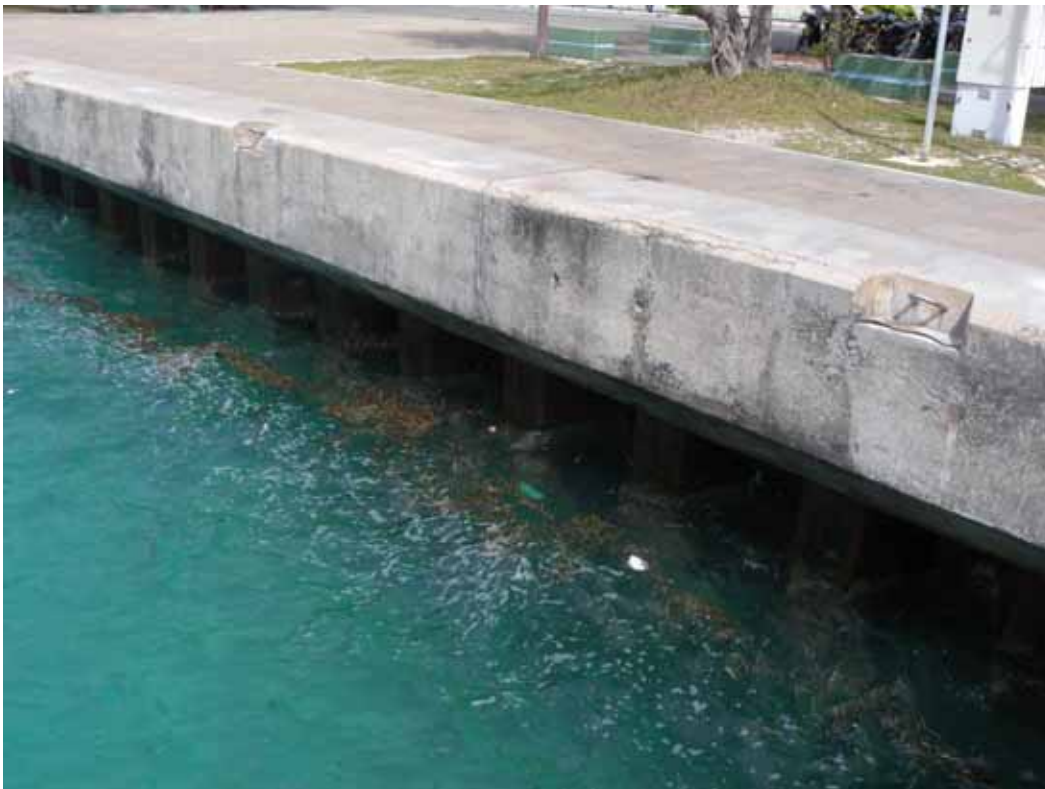
Figure 4.30 A modern quay wall in Hulhumale' constructed from sheet piles and concrete
