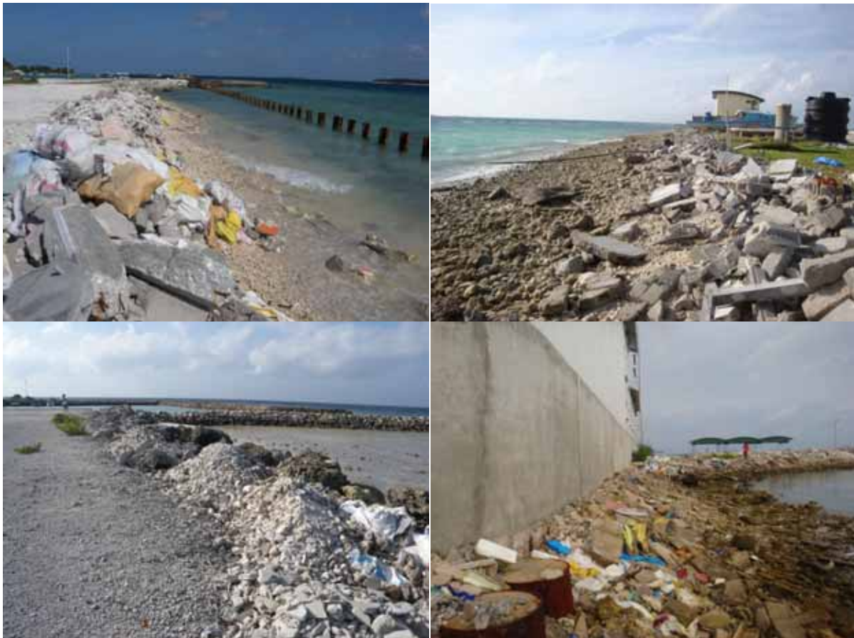
Figure 5.17 Use of both construction debris to protect properties from flooding in S. Feydhoo
