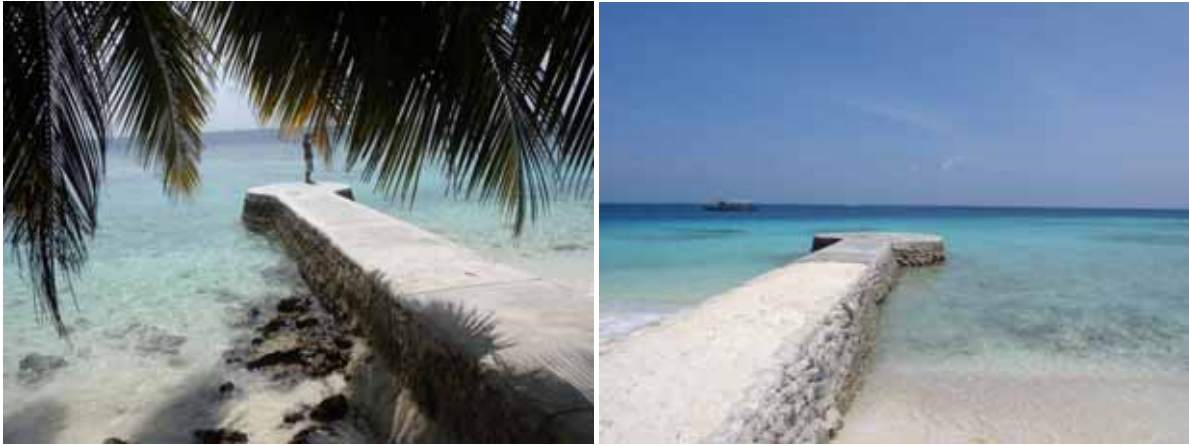
Figure 4.26: Sand cement bag and coral mound groynes in Sun Island Resort
