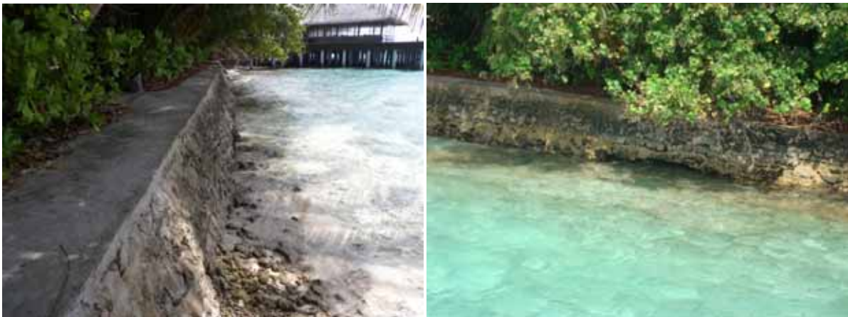
Figure 4.7: Examples of Sewall structures: semi-plastered coral mound seawall in Boduhithi
