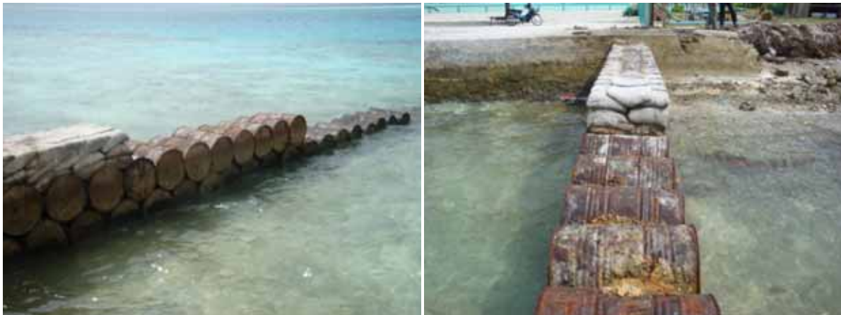
Figure 4.28 Groynes constructed concrete filled empty oil barrels in M. Maduvvari
