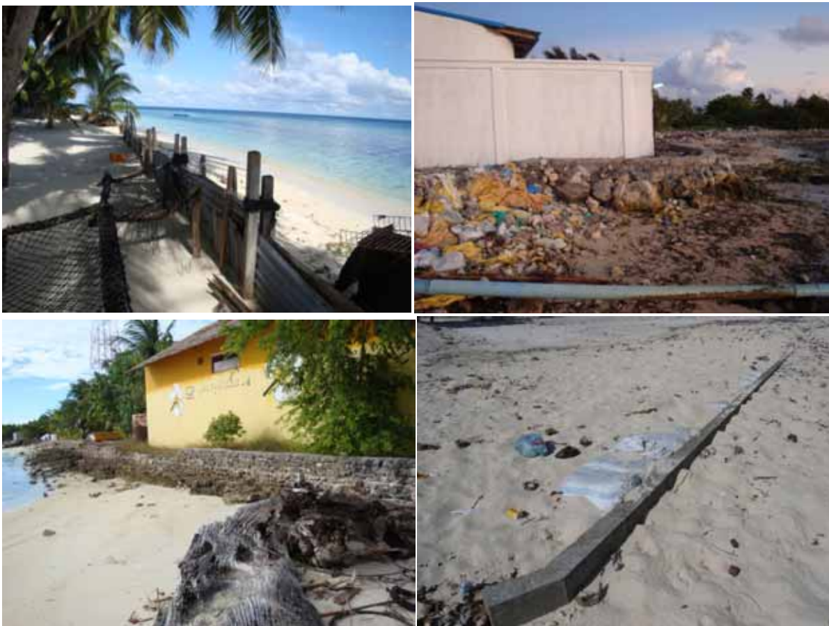
Figure 4.14: Adhoc seawalls in (clockwise from left) GA. Dhevvdhoo , GDH Thinadhoo, GA Kolamaafushi and B. Eydhafushi
