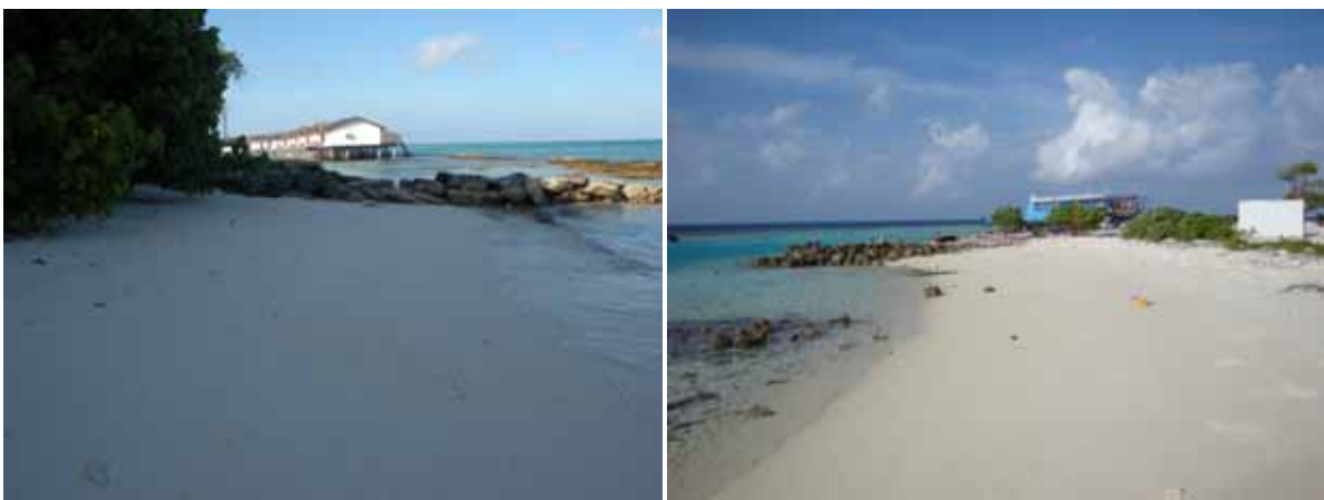
Figure 4.27 Groynes constructed from coral rubble in B. Reethi beach and AA Bodufolhudhoo
