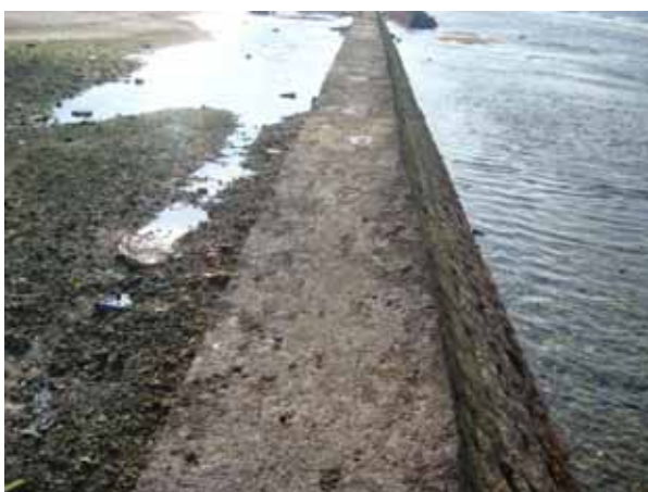
Figure 4.18: Generic fore-shore break water design – Sand Cement bags in AA Bodufolhudhoo and Neykurendhoo
