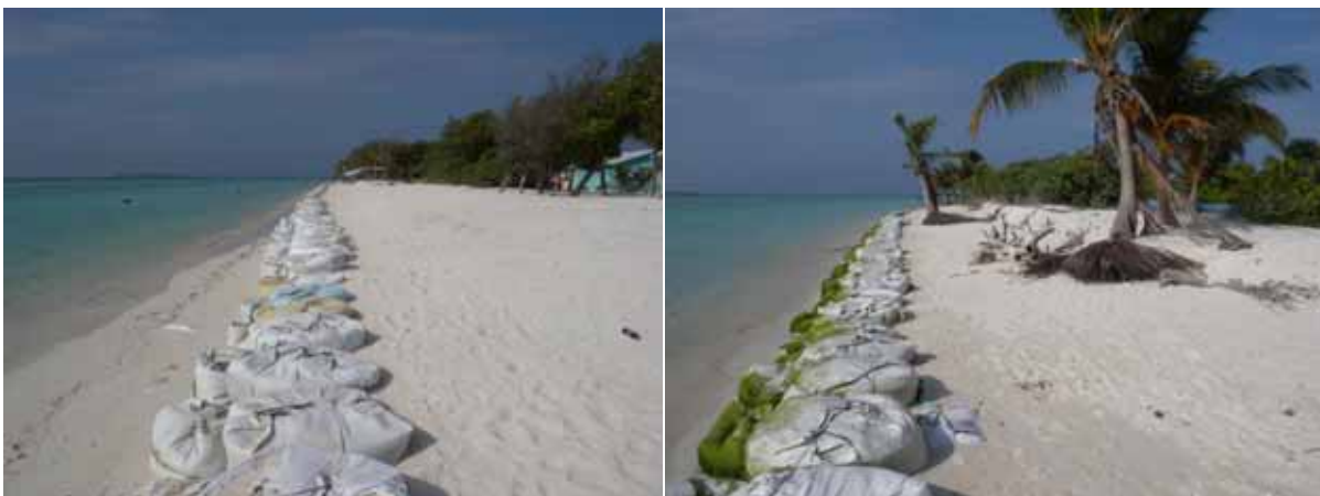
Figure 4.12: Examples of Sewall structures: 'Jumbo bags' in R. Dhuvaaafaru
