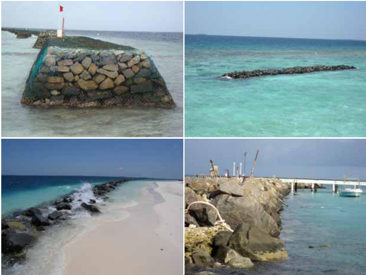
Figure 4.18: Generic fore-shore break water design – Sand Cement bags in AA Bodufolhudhoo and Neykurendhoo
