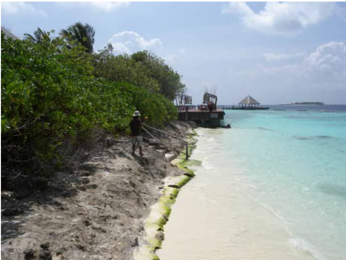
Figure 4.23: Generic revetment design – Rubble slope with concrete plastering in K. Boduhithi
