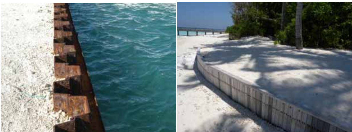
Figure 4.10: Examples of Sewall structures: Sheet piles in Fun Island Resort and wooden piles in Irufushi Resort
