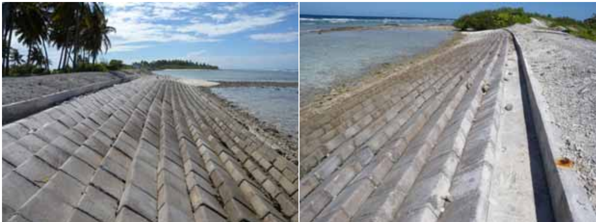
Figure 4.21: Generic revetment design – Interlocking concrete blocks in S. Hithadhoo
