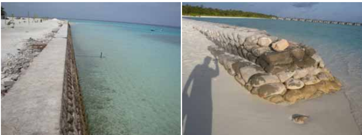
Figure 4.10: Examples of Sewall structures: Sheet piles in Fun Island Resort and wooden piles in Irufushi Resort
