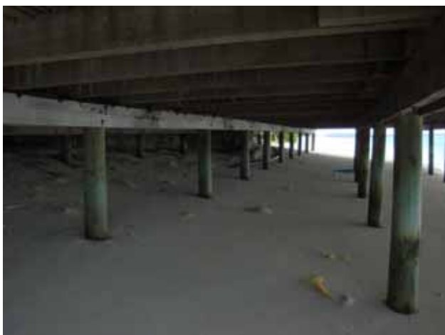
Figure 5.22 Use of stilts and retaining walls in Dh. Vilu Reef Resort
