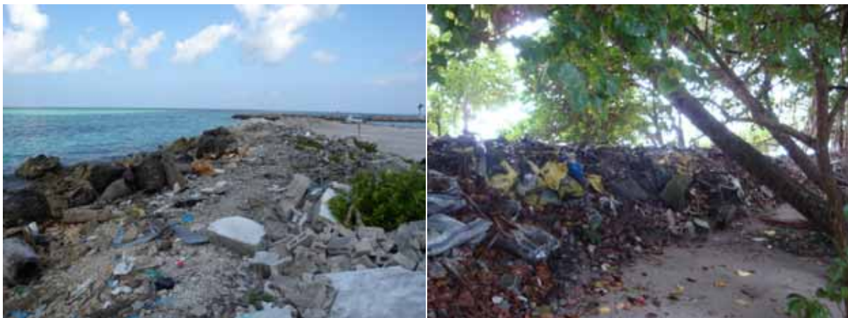
Figure 5.19 Use of both construction debris and green waste as an adaptation measure against erosion in HDh. Hanimaadhoo and V. Keyodhoo
