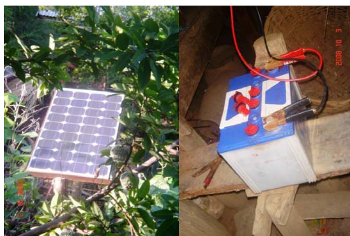
3. Recharging battery with electricity generated by solar panels, Sakawar SRG in Moe Nan Kyin village in Kyaukpadaung
