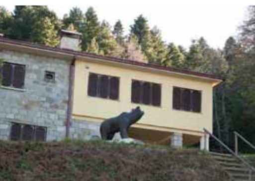
Information Center in National Park Pelister photo: Lj. Stefanov
