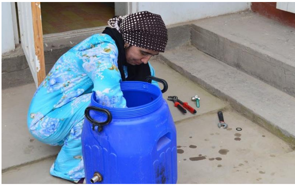
UNDP Photo: Savri Badalova prepares a water tank for the solar water heater system during the workshop.
