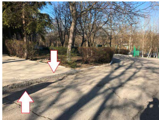
Concrete surface, curb of about 15 cm
