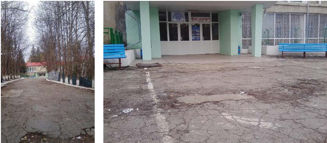
Broken parts of sidewalk and road, asphalted surface, lack of tactile pavement or contrasting marking
