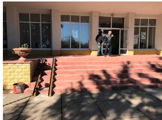
2020 – Ramp improvised out of metal rails
