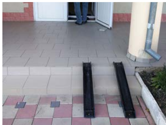
2020 - Ramp improvised out of metal rails
