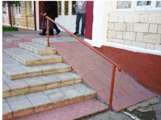
2020 – Support bar on steep ramp (34°)
