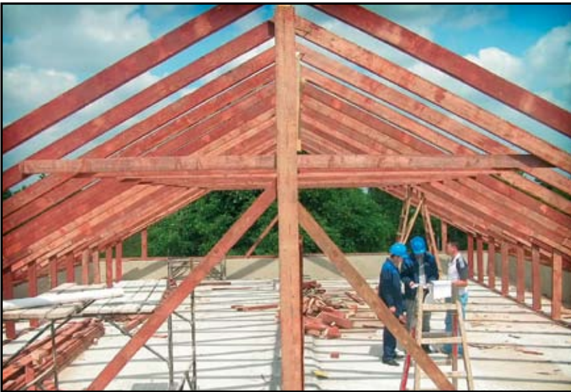
In Edinet the roof of the future Centre was rebuilt anew.
