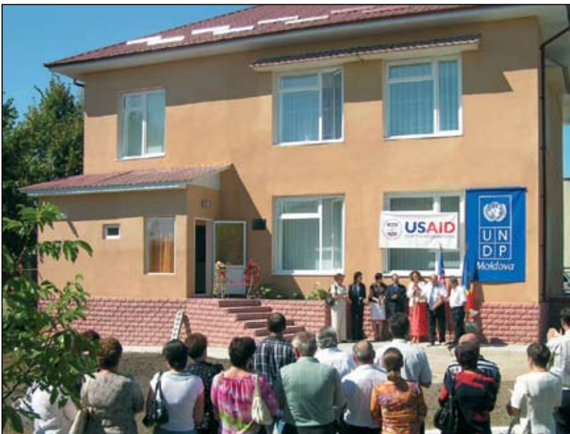
Before becoming ARIADNA Maternal Centre, this place was an abandoned wing of a kindergarten from Drochia.
