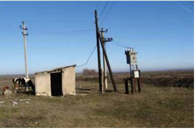
In Crasnoe, the protection zone around the well was restored and electrical power equipment, including a transformer and an automated pump, were installed as part of the water supply project. Now, the water runs through a pipeline, and thus, life goes on.
