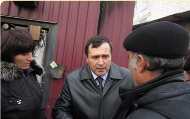
Biomass boiler in School of Antonesti village
