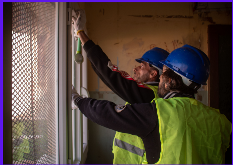
Ongoing work to renovate Al Hakh Revolution School
