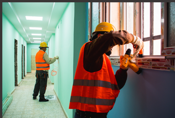
Ongoing work to renovate the Diabetes Facility at Bani Walid Hospital
