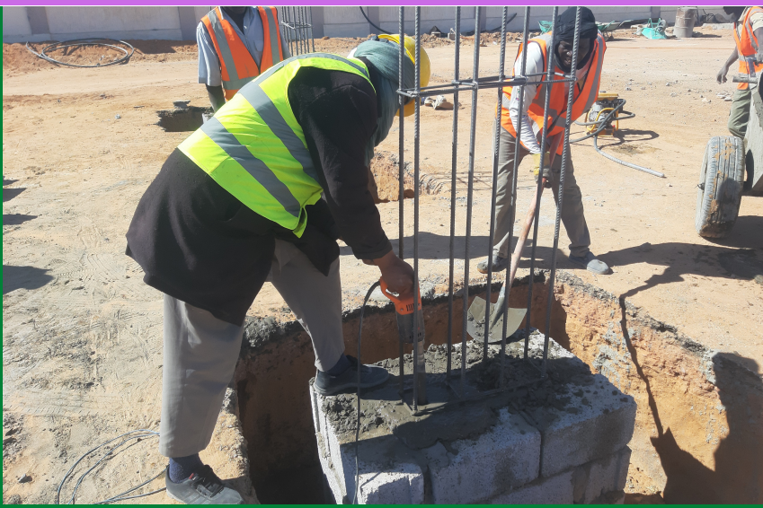
Ongoing work to build the National Legal Training Center
