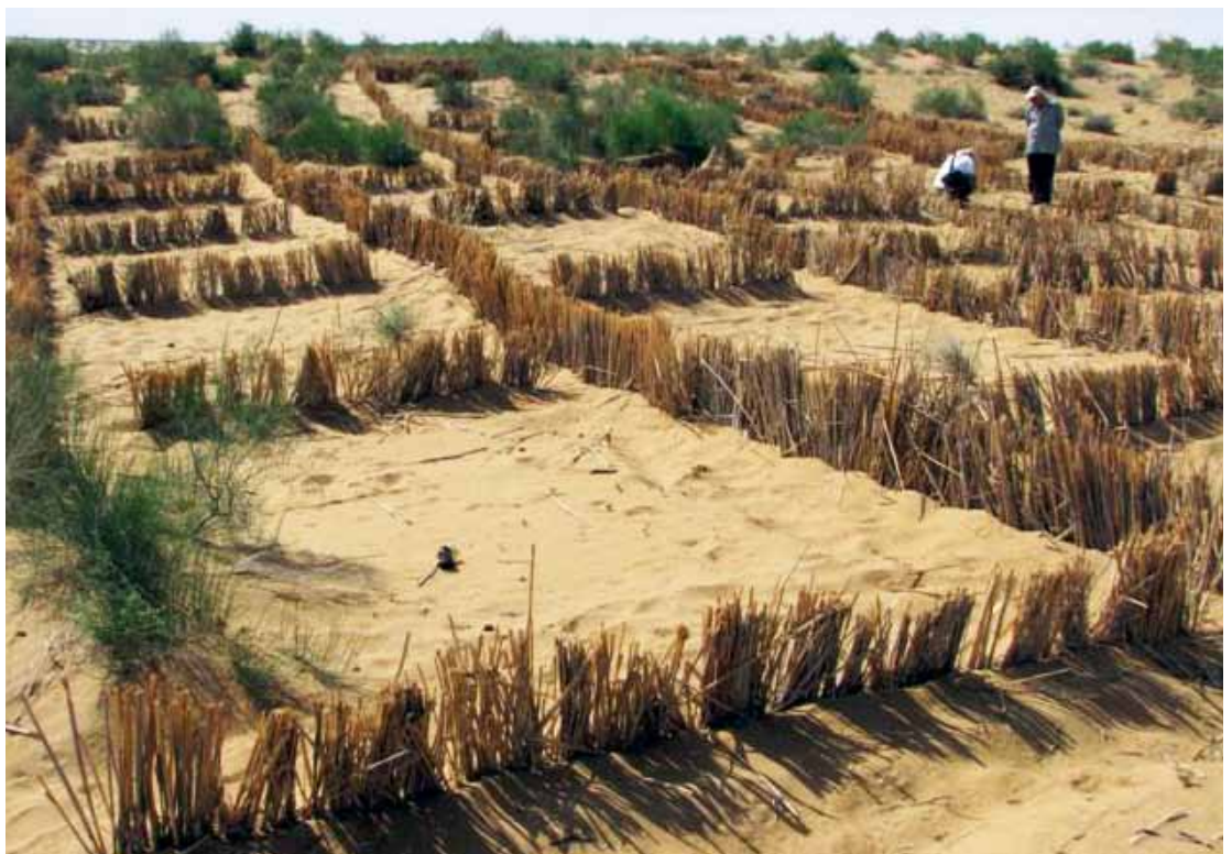
Barriers installed in Uzbekistan as part of an anti-desertification effort funded by UNDP, GEF and the Government.
