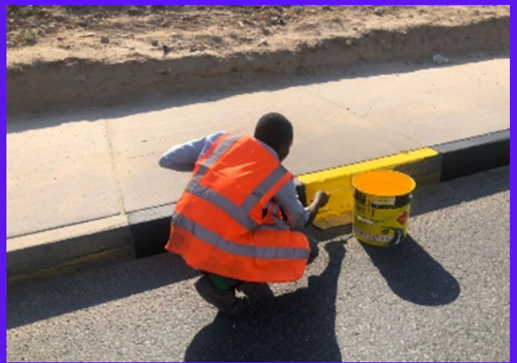
Ongoing work to renovate the second ring road in Tripoli, November 2021
