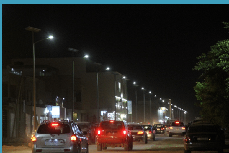
One of the previously unlit streets in Benghazi.
