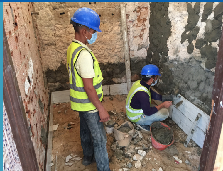
Ongoing work to renovate Al Kikhia Cultural House
