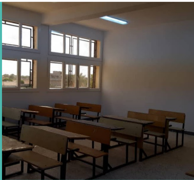
One of the already completed classrooms at Al Yarmouk School
