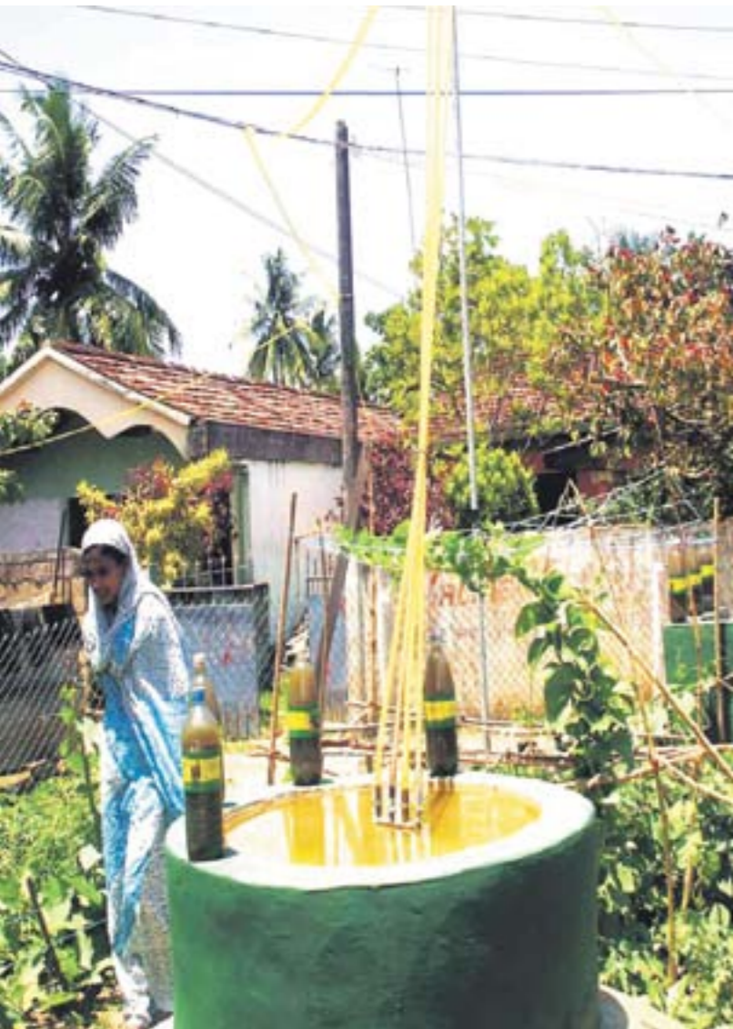
A community biogas unit
