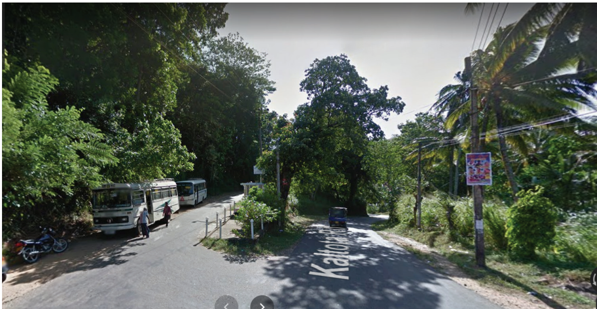
Figure 7: 33kV primary distribution line running through the Balangoda site.
