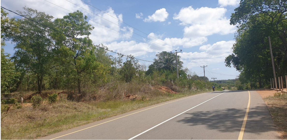
Figure 6: 33kV primary distribution line running through the Thanamalvila site.
