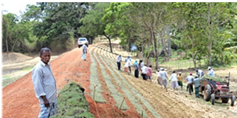
Community participation in turfing the earth dam to prevent erosion
