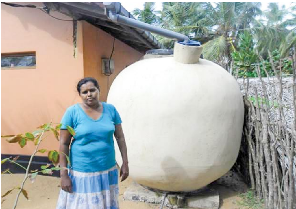
Rainwater harvesting tank in village household
