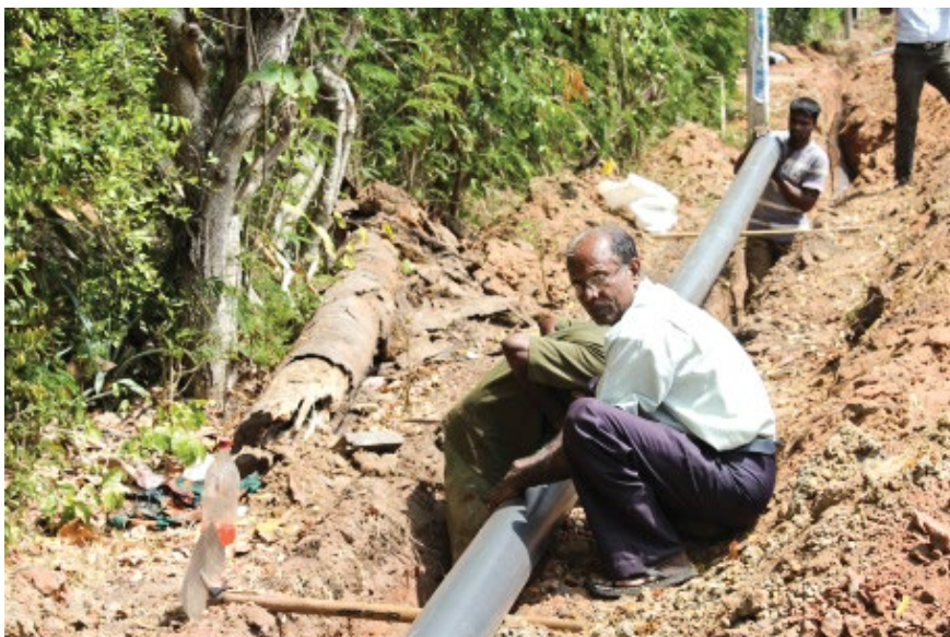
Laying out pipes
