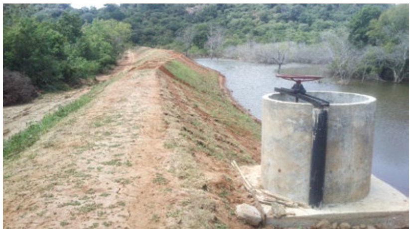
The completed tank
