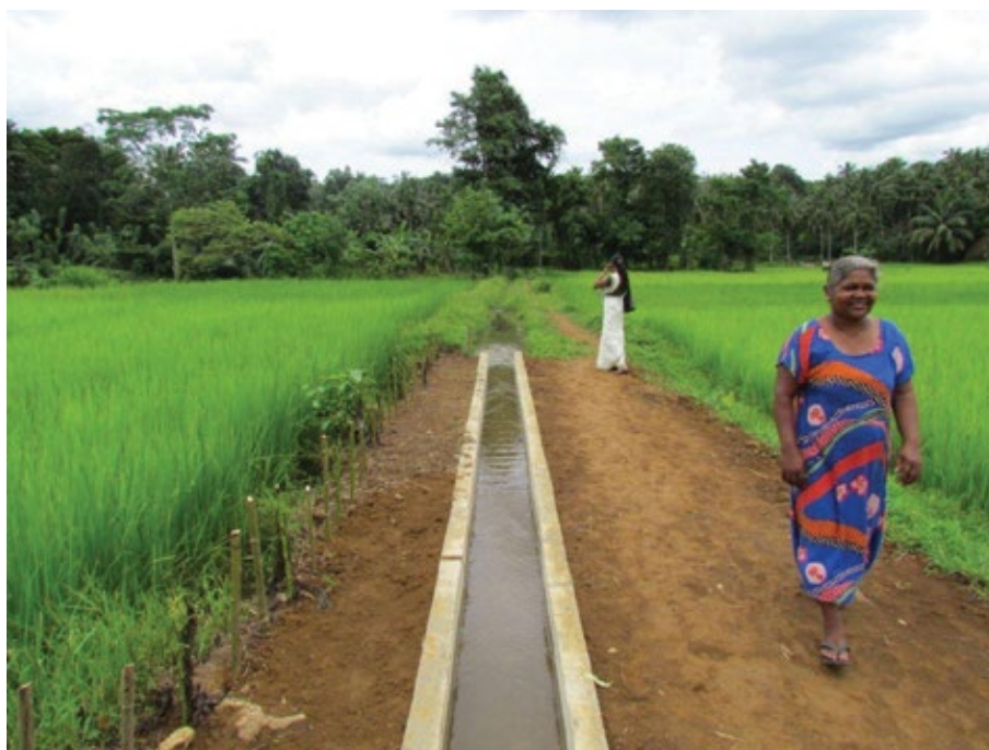
Upgraded water channels bringing water during extended dry seasons and also help reduce flooding during the rainy season
