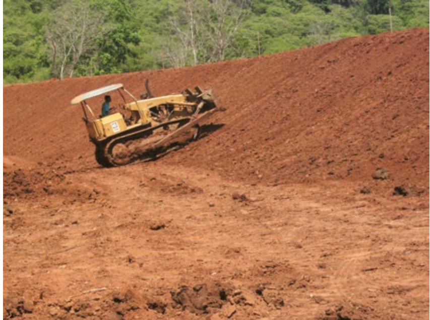
Construction of the tank
