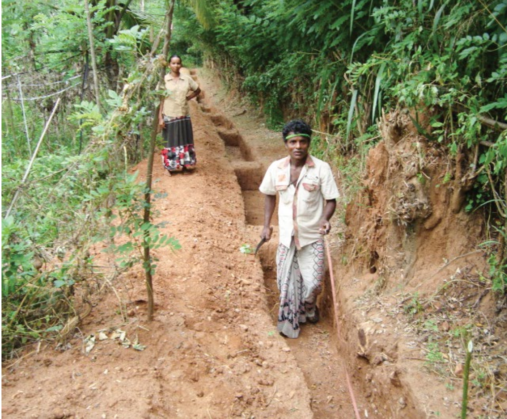
Erecting stone bunds in gardens
