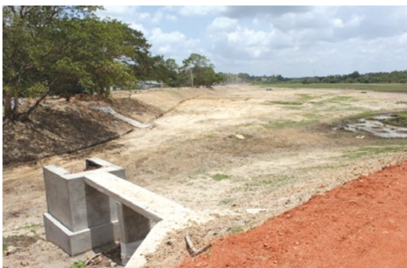
The village reservoir after earthwork and dredging
