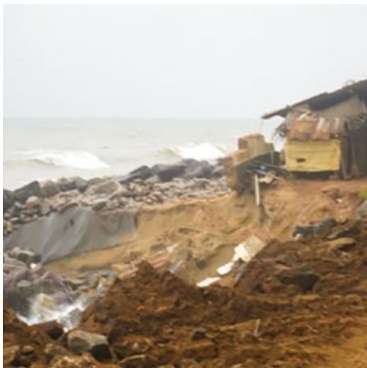
Coastal erosion in Barudelpola village
