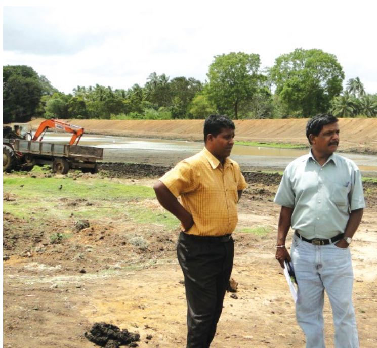
Government technical officers supervising the dredging of the reservoir
