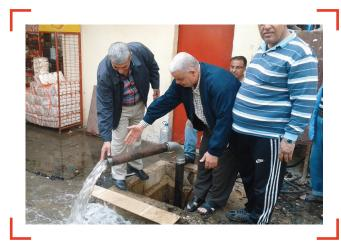
Rehabilitation works included installing a new pump and pipes after excavating the concrete road from the well to the main pipe as well as installing the necessary electrical boards for the pump. "As we have been waiting a long time for this intervention, the popular committee established an electrical room to preserve the new equipment provided by UNDP from environmental and human damage," explains Anbour.
