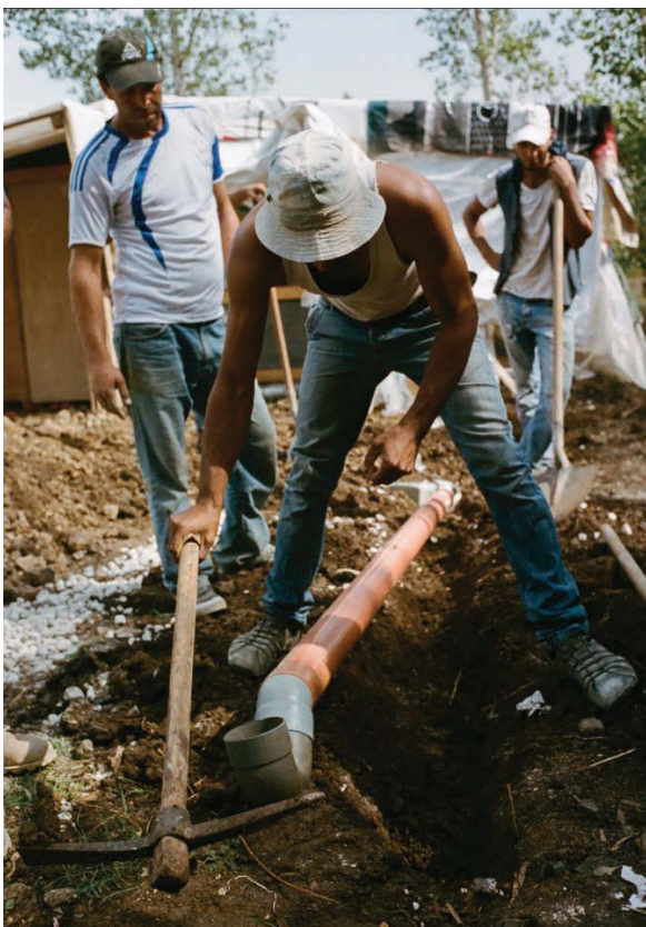
Construction of latrines.
