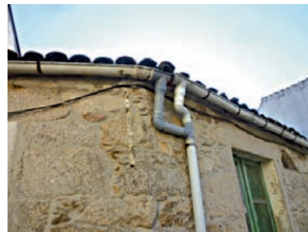
Fig. 20 Detail of a common Downspout
