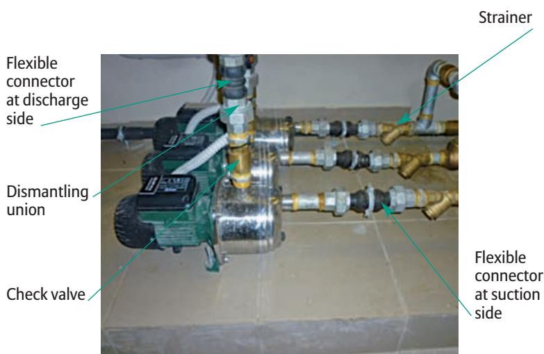
Fig. 39 Booster pump connection details
