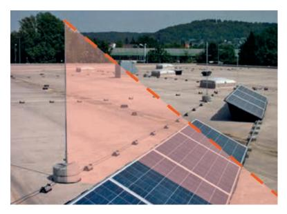
Figure 30 - Angle method example (Source: Dehn)
