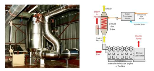
Figure 39: Exhaust gas boiler
