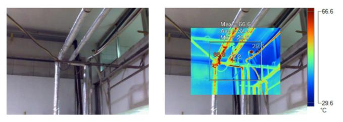
Figure 30: Example of poor insulation in steam pipes
