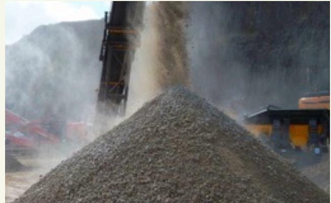
Figure 6: Use of mechanical sprayer
