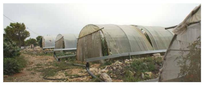
Pilot installation of a greenhouse rainwater harvesting system in Kfarmashoun — Byblos (Photo from V. Kabakian)
