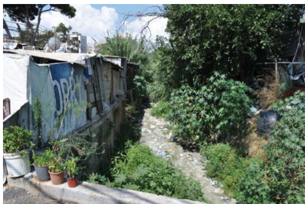
Figure 7-8 Informal Makeshift Constructions on Nahr el Ghadir, Kfarchima Photo Credit: Yazigi Atelier, 2020
