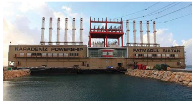
Figure 9-16 Fatmagul Power Ship at Jiyeh Power Plant Photo Credit: Karpower
