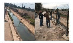
In the upper part of Qasmieh, considered the largest Palestinian Gathering in Lebanon, UNDP has also installed a 150 meter storm water network and built two retaining walls for safety, before paving the affected roads.
