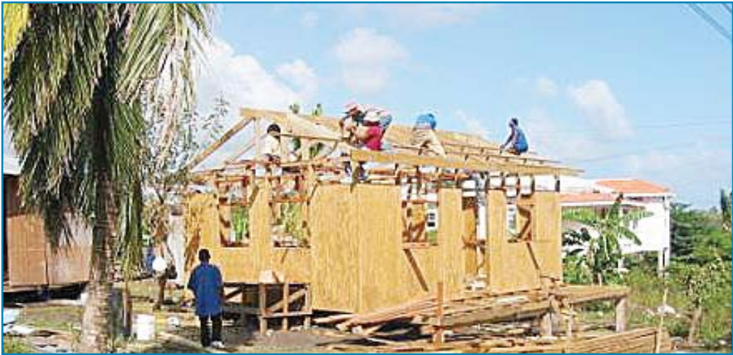
Construction of low income house
