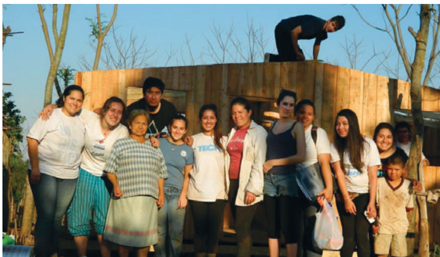
In Paraguay, 500 national and 1,200 Chilean volunteers helped to build over 250 houses with funding and knowledge sharing from the 'Chile Fund Against Hunger and Poverty', a UNDP-Government of Chile South-South Cooperation partnership.
