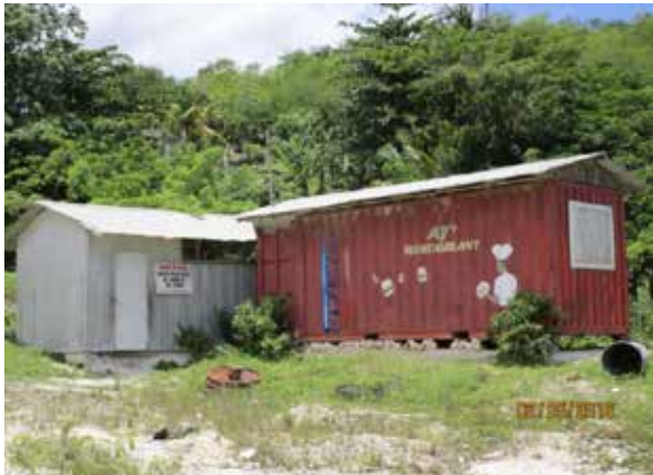
Group 3 staff facilities
