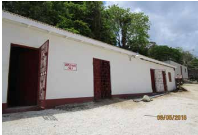
Photo 5 Good staff facilities at Group 4 quarry, Trelawny Parish
