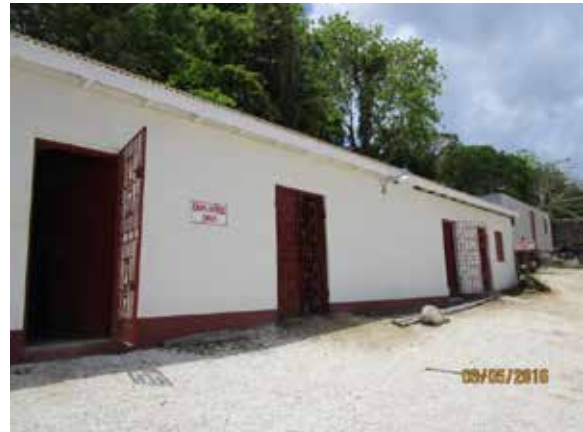
Group 4 staff facilities
