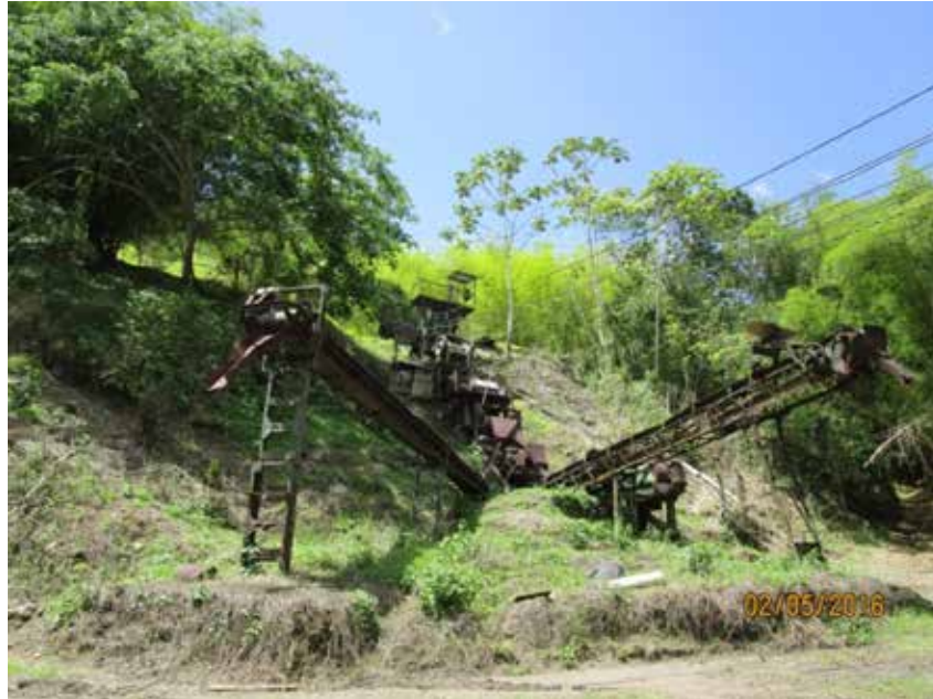
Photo 9 Old Conveyor Equipment Requiring Upgrade, St. James
