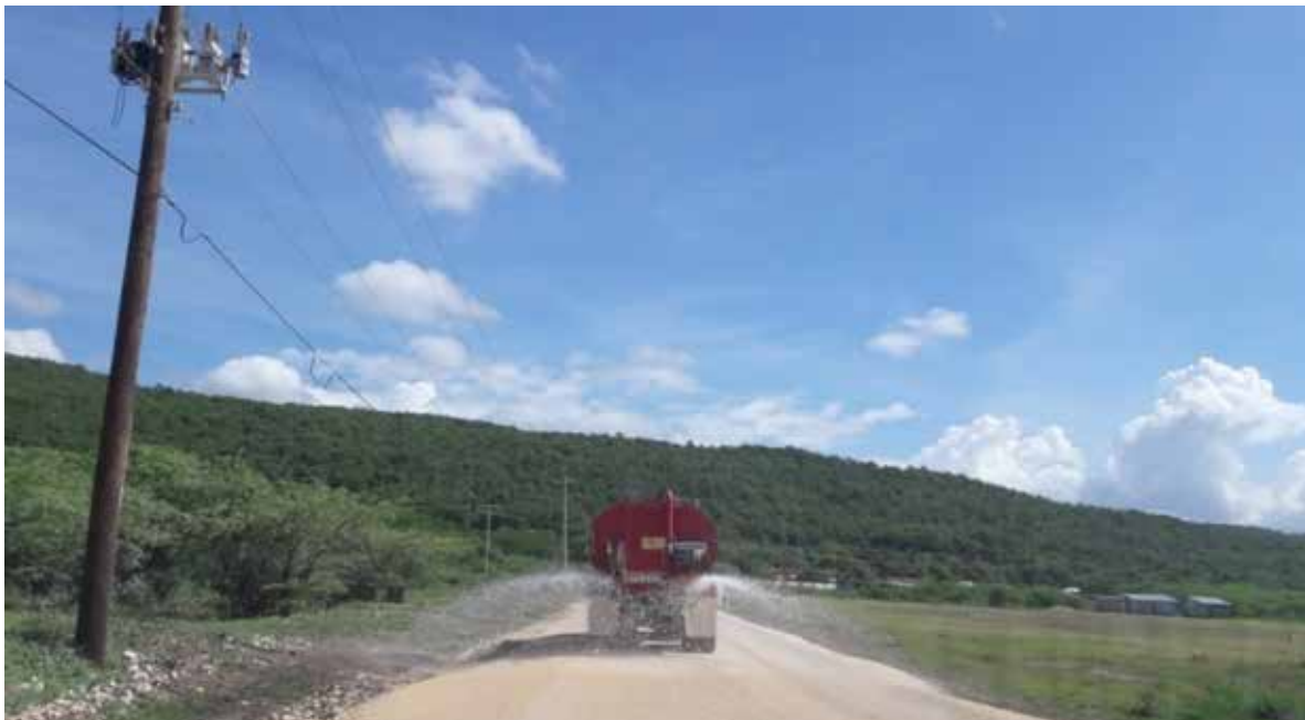
Photo 35 Dust suppression - water spraying truck on Quarry access road
