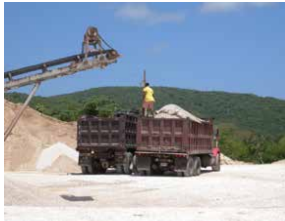
Photo 27 Quarry worker with no PPE, exhibiting dangerous behaviour also
