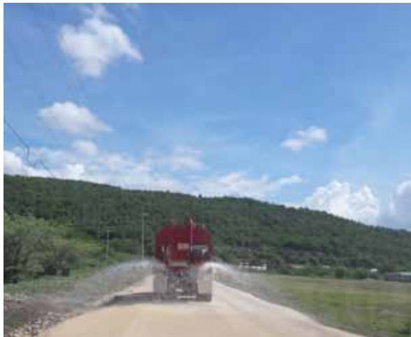
Sprinkler truck suppressing dust on Quarry haulage road, May 2017
