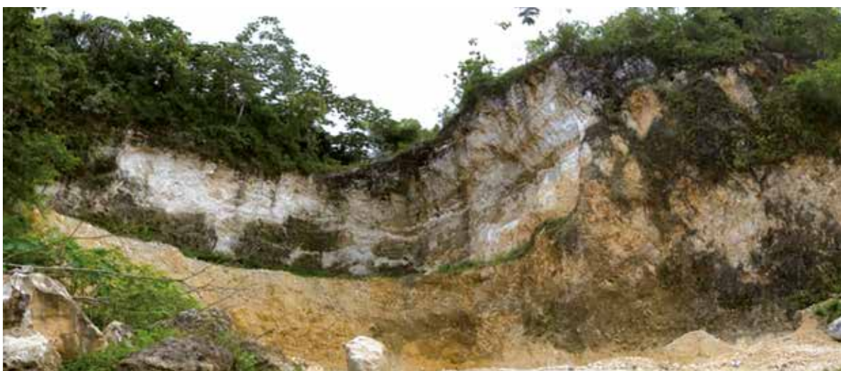
Photo 25 Ripping of 'soft' material from the base of the quarry face leads to dangerously unstable quarry overhangs
