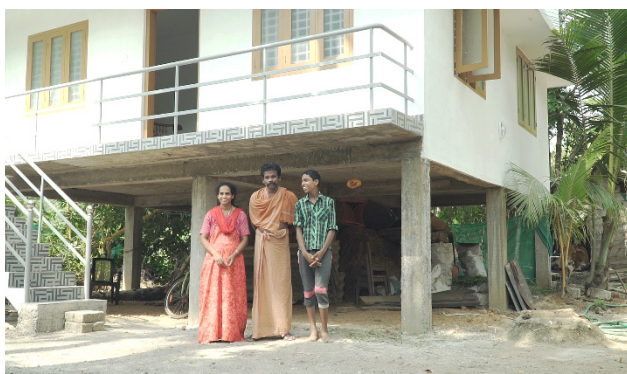
Photo 1: Flood Resilient House Reconstruction on Stilts
