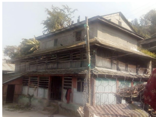
Photo 2: 70 year old House Retrofitted
