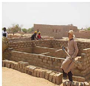
School construction in Albarkayzé
