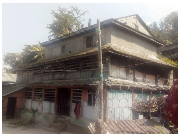
Photo 2: 70 year old House Retrofitted
