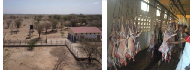
Aerial view of the newly completed Kakuma Slaughter House And Meat being processed at the Kakuma Slaughter House: the facility has provided hygienic space for handling meat. The facility serves both local (host) population and refugees in Kakuma and Kalobeyei Refugee Camps.
