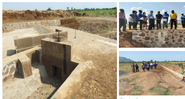
The weir and canal rehabilitated
