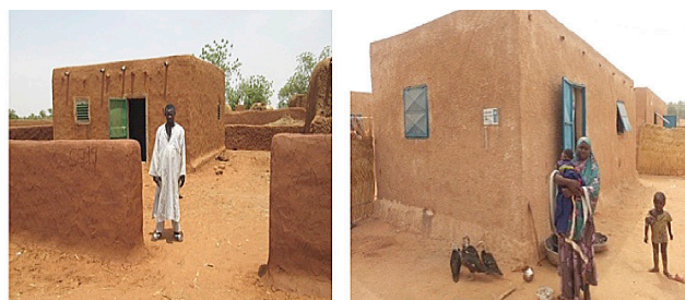
House "built back better" with the local material in Bantali
