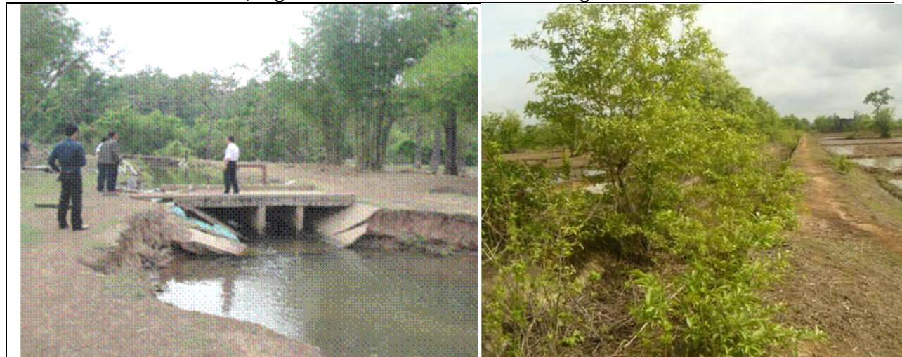
Picture 9: Culvert over an irrigation channel is unstable due to flash flood scouring the channel banks downstream from the culvert. The culvert foundation needs to be tied back and channel re-lined with concrete.
