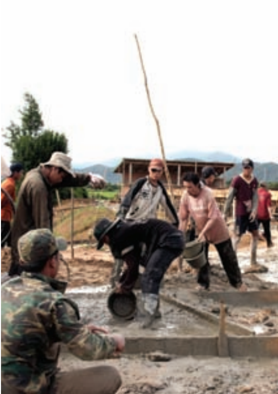
Safety in the workplace can ensure decent work
