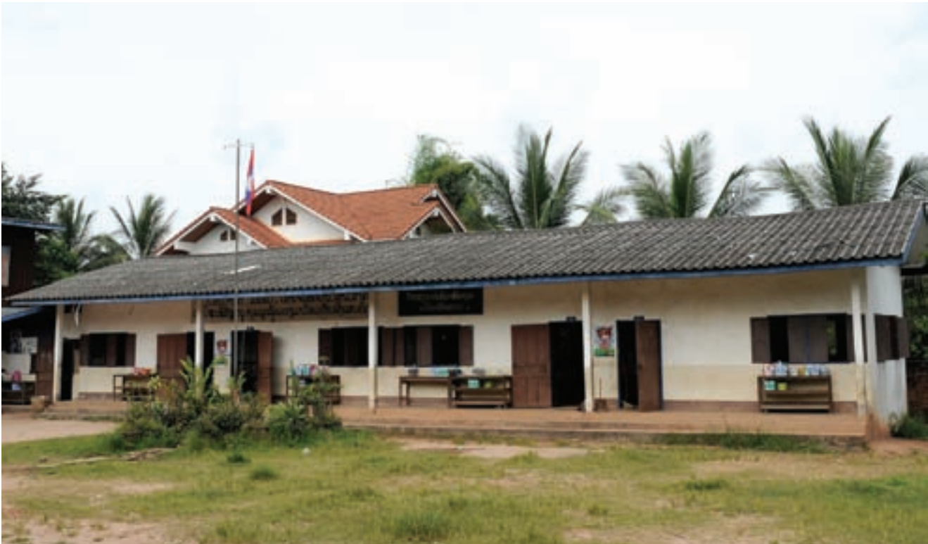
A prerequisite for good learning is the provision of basic infrastructure for rural schools
