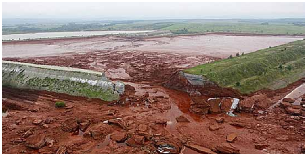
Photo 3. Tailing dam collapse in Hungary 2010.
