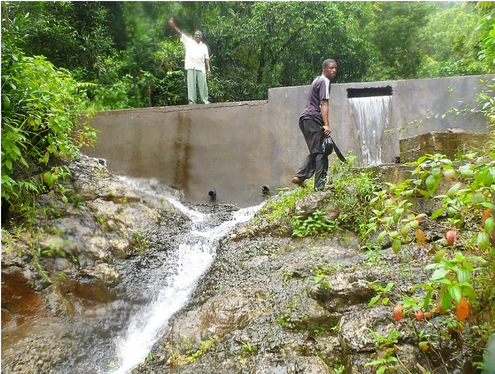
Figure 6 Typical river intake structure.
