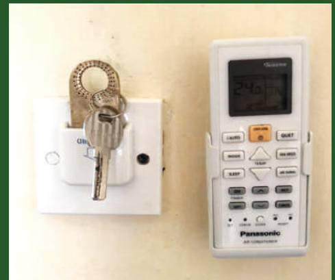
Example of EMS in a hotel using a room key to control electricity
