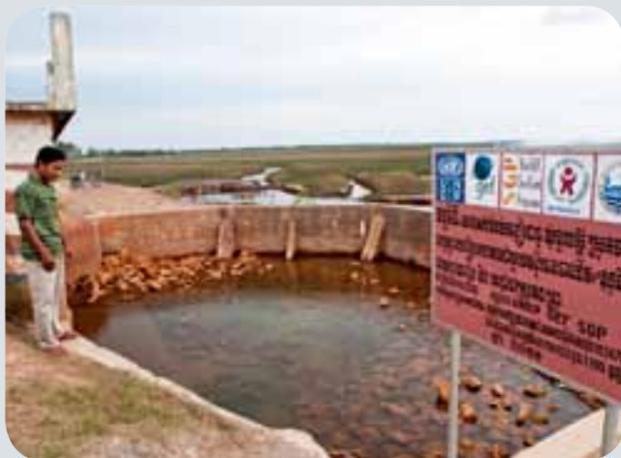
A water dam built with support from a joint project of UNDP and GEF allows residents in Kampong Sdey commune, Svay Rieng province, to improve food security by growing rice two times, instead of one, per season.
