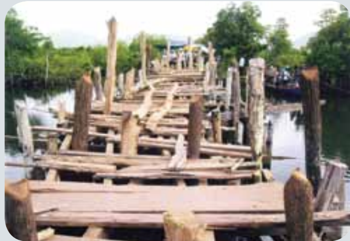
The old bridge at Kampong Sdam river in Koh Kong province.
