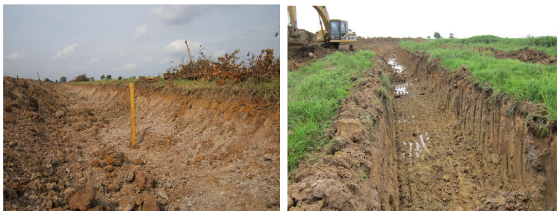
Figure 3: Canal rehabilitated for irrigation and flood drainage in the target area
