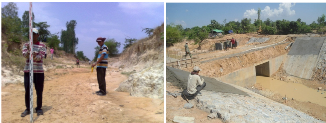
Figure 4: Spillway constructed to keep water in the canal and to bring more water to the lake reservoir in the target area
