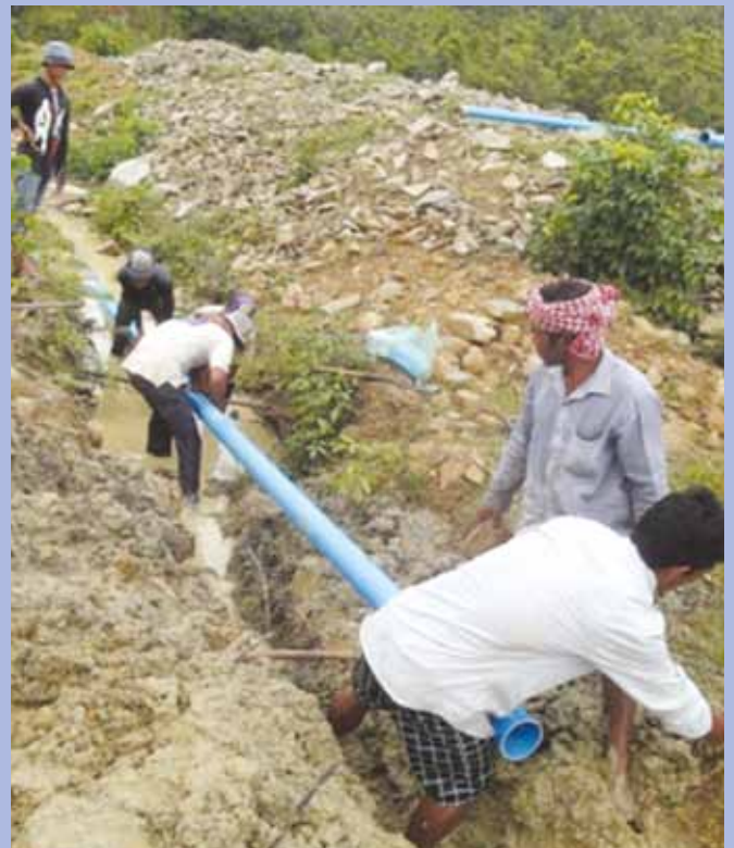
Labourers installing the pipe network from the water reservoir to residential areas in Kraing Serei village
