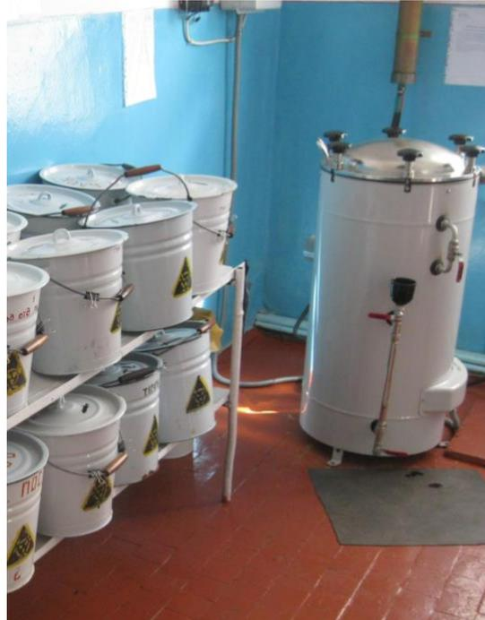
**Figure 4. Autoclave BK-75 and microwave oven at medical waste decontamination points in health care organizations of the Kyrgyz Republic**
