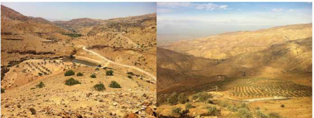
Figure 4.4: Photos for Tel Dahab conversion dam (left), Homrt Aldyghami near Tel Dahab conversion dam (left) and a rainfed olive farm that replaced annual crops near Zarqa River in Sbihi as an adaptation measure to climate change (Naser Almanaseer, May 15th 2014)
