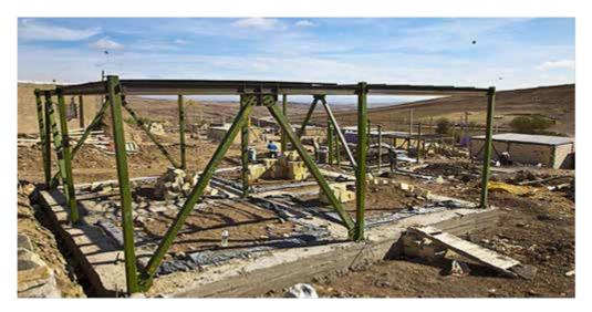
Bolt and nut steel frames (steel frames are factory made)
