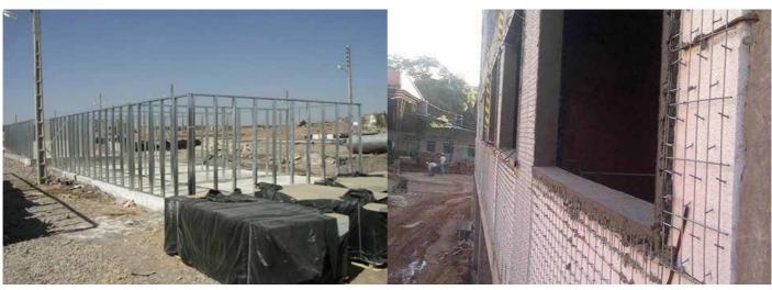
Light Steel Frame – LSF (factory made elements but labor intensive at the site)
