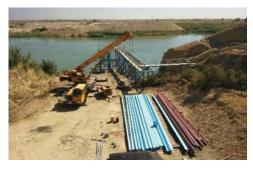
Excavator at the intake of Tikrit water pumping station to repair the water network
