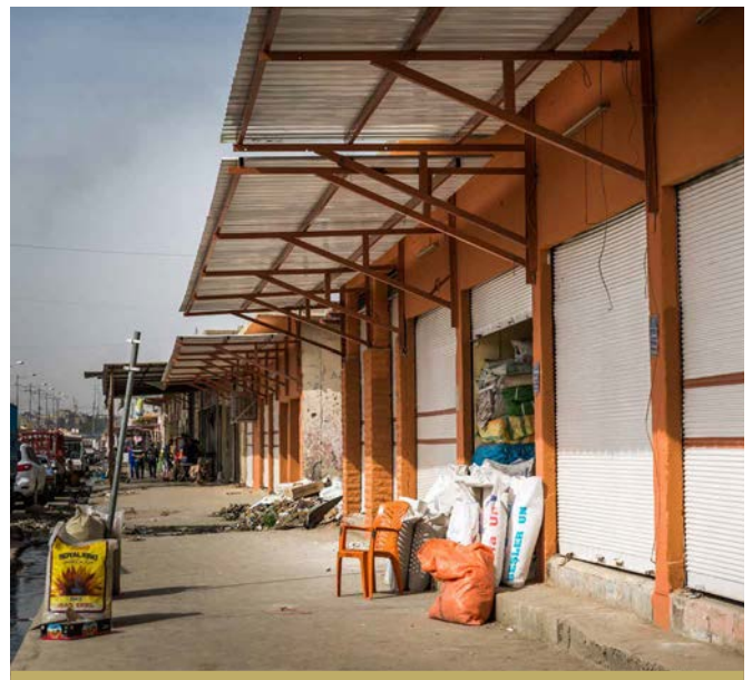
A STALL IN THE YABESAT MARKET IN WEST MOSUL, BEFORE AND AFTER THE MARKET'S REHABILITATION BY FFS. TOGETHER WITH THE 300-STALL VEGETABLE MARKET, THE REHABILITATION OF THE YABESAT MARKET ALLOWS SOME 1,000 MERCHANTS TO RETURN TO 270 STALLS AND SHOPS AND PROVIDE FRESH FOOD, GRAINS AND SEEDS TO PEOPLE. ©UNDP IRAQ/CLAIRE THOMAS
