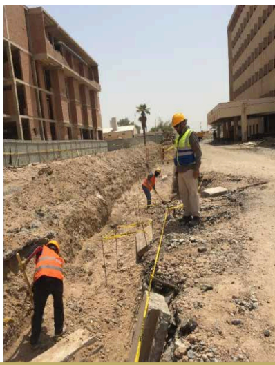
TRENCHES ARE DUG TO INSTALL CABLES ON THE SITE OF THE TIKRIT TEACHING HOSPITAL. THE REHABILITATION OF THE ENTIRE TTH COMPLEX IS THE LARGEST FFS PROJECT, JOINTLY IMPLEMENTED BY FFIS AND FFES, WITH A TOTAL BUDGET OF USD 40,000,000 AND NUMEROUS SUB-COMPONENTS OF THE MAIN REHABILITATION PROJECT.
