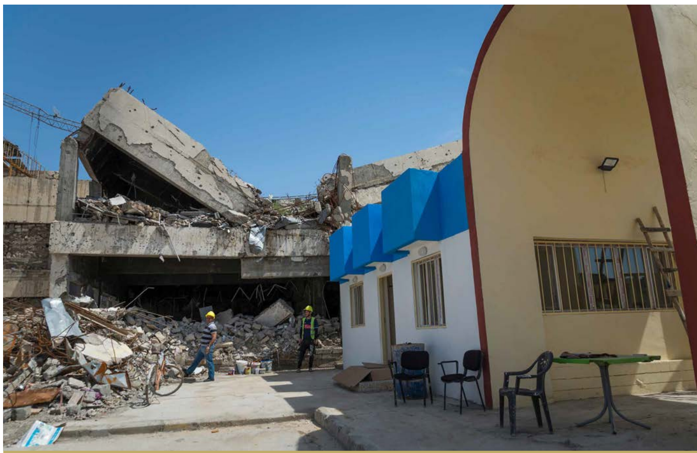
THE AL-JAMHOURIYA POLICE STATION AT THE AL SHIFAA HOSPITAL COMPLEX IN WEST MOSUL, PRIOR TO ITS REHABILITATION BY FFS. ©UNDP IRAQ/CLAIRE THOMAS
