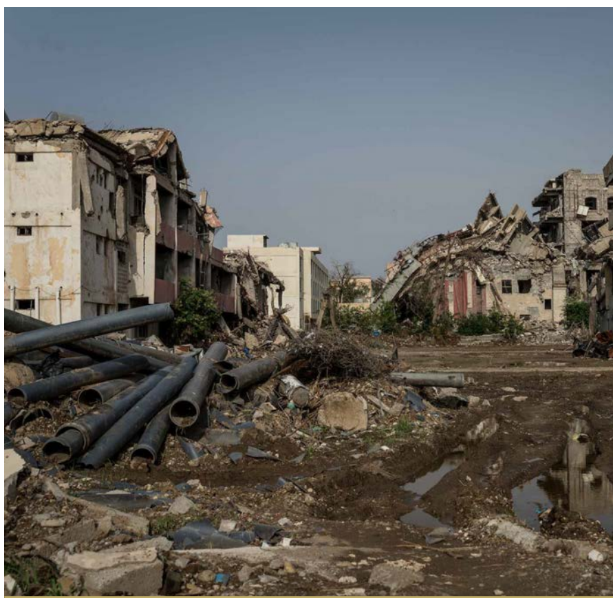
DESTROYED BUILDINGS AT THE MOSUL UNIVERSITY. PREPARATORY WORKS FOR THE REHABILITATION OF MOSUL UNIVERSITY ARE ONGOING. DURING THE REPORTING PERIOD, A MAPPING EXERCISE FOR MOSUL UNIVERSITY WAS UNDERTAKEN IN ORDER TO PRIORITIZE PORTIONS OF THE CAMPUS FOR REHABILITATION AND COORDINATE THE REHABILITATION PROCESSES BETWEEN THE ACTORS TAKING PART. ©UNDP IRAQ/CLAIRE THOMAS
