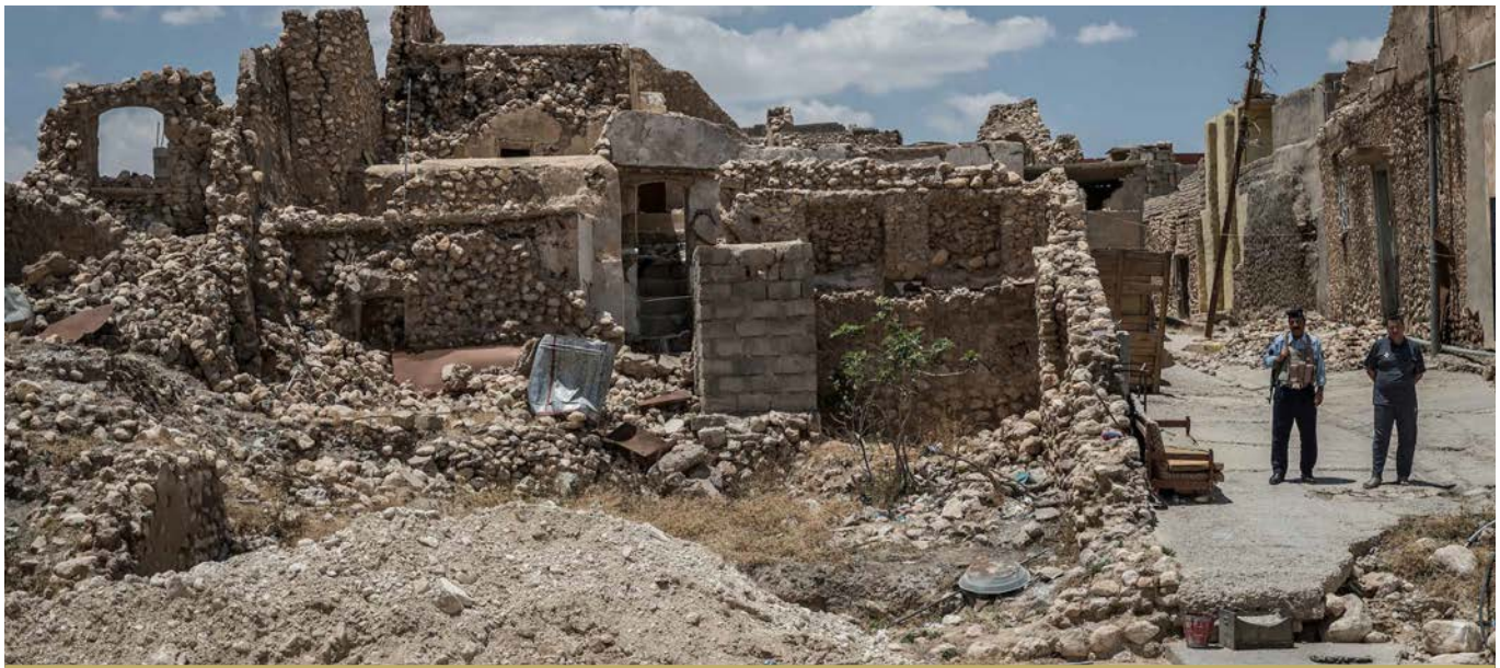
THE RUINS OF THE HISTORIC CENTRE OF SINJAR CITY. ©UNDP IRAQ/CLAIRE THOMAS
