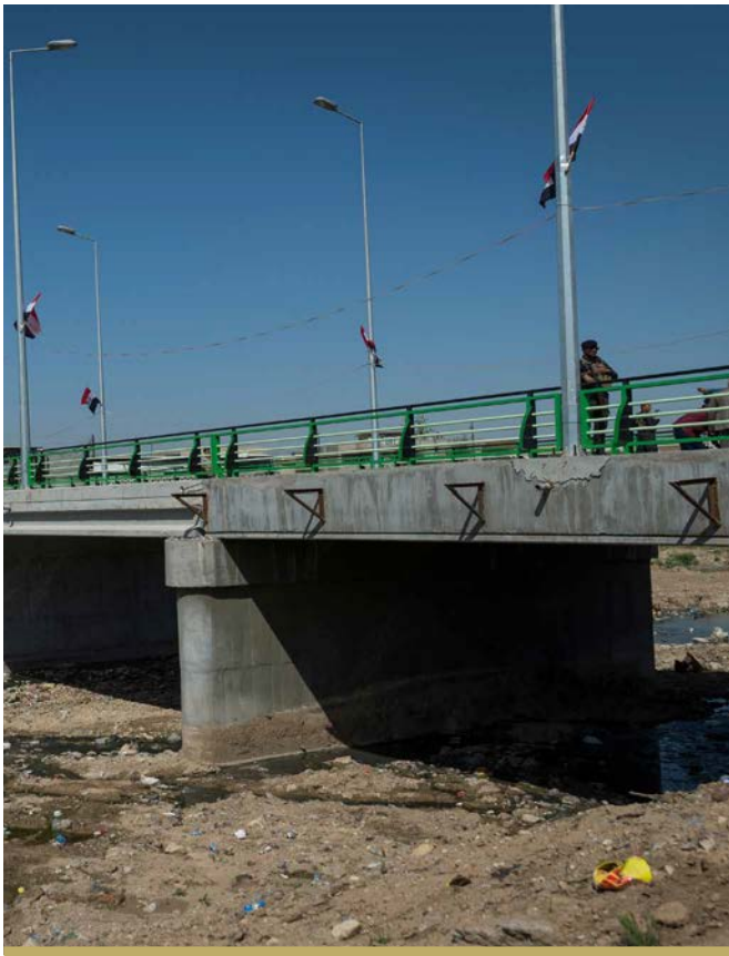
THE COMPLETED SAYEDATEE AL JAMILA BRIDGE IN EAST MOSUL, WHICH WAS CEREMONIALLY OPENED DURING Q2. ©UNDP IRAQ/CLAIRE THOMAS
