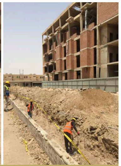
TRENCHES ARE DUG TO INSTALL CABLES ON THE SITE OF THE TIKRIT TEACHING HOSPITAL. THE REHABILITATION OF THE ENTIRE TTH COMPLEX IS THE LARGEST FFS PROJECT, JOINTLY IMPLEMENTED BY FFIS AND FFES, WITH A TOTAL BUDGET OF USD 40,000,000 AND NUMEROUS SUB-COMPONENTS OF THE MAIN REHABILITATION PROJECT.
