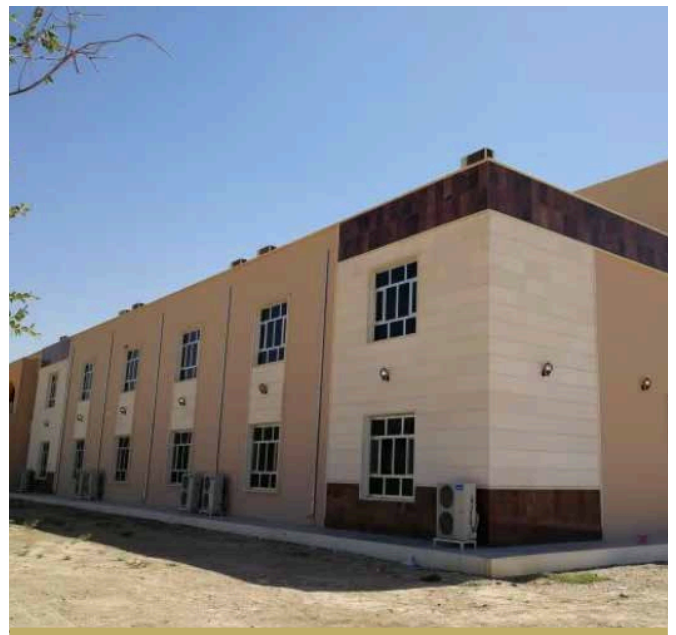
WORK ON THE CIVIL ENGINEERING DEPARTMENT OF THE COLLEGE OF ENGINEERING WAS ALMOST COMPLETE BY THE END OF THE REPORTING PERIOD AND IS EXPECTED TO BE FINISHED EARLY IN Q3.
