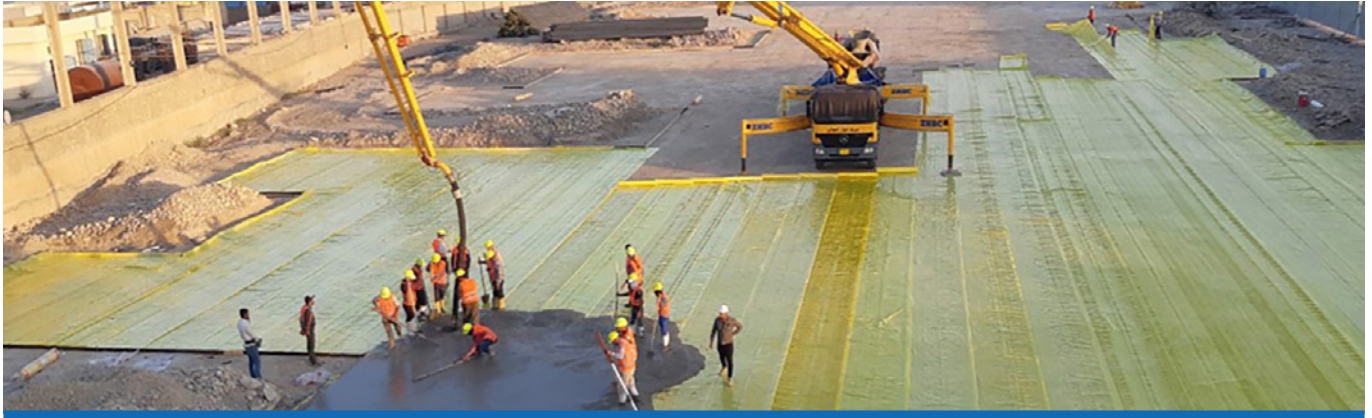
Work is ongoing at the West Mosul High Court Complex.
