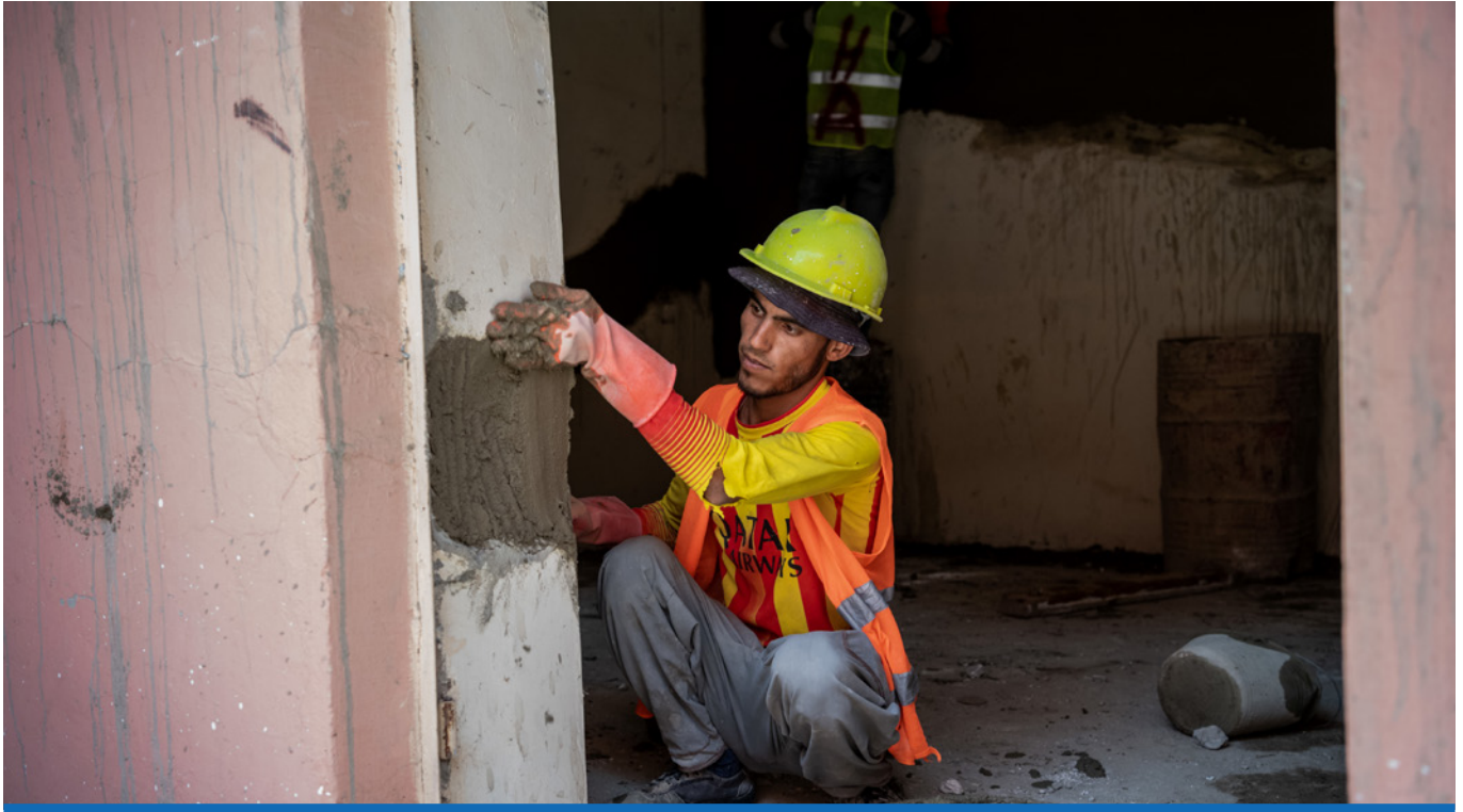
Work is ongoing to support the rehabilitation of houses in Batnaya.
