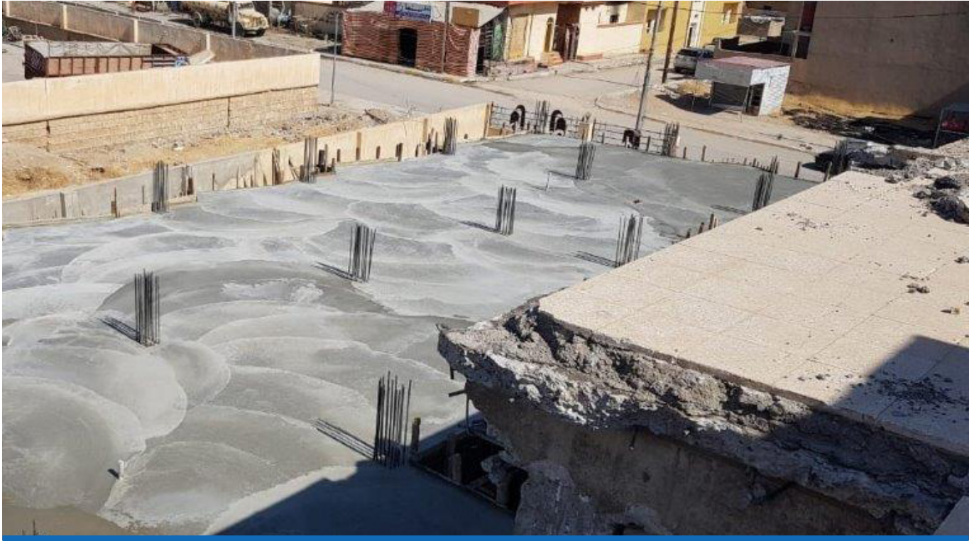
The Sinjar Municipality Building was underway during the reporting period.
