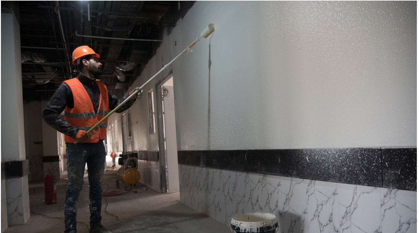
Work is ongoing at the Ramadi Maternity Hospital.
