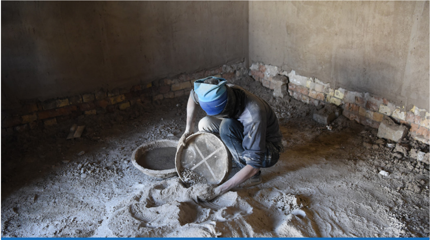
A worker plasters a wall in a home in Ramadi.
