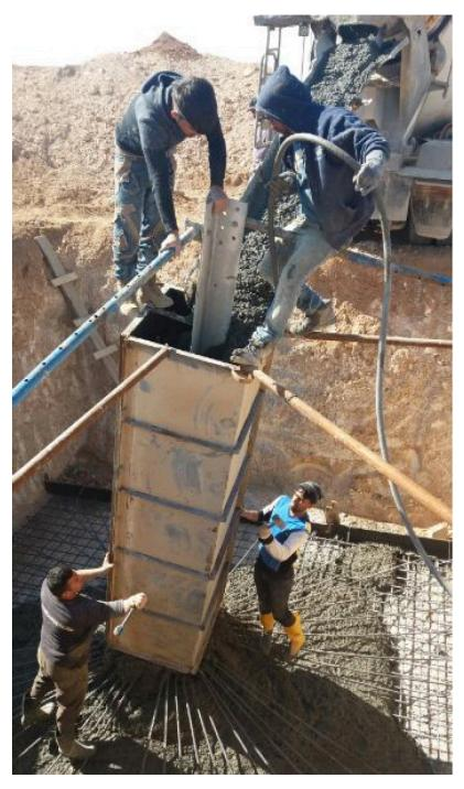
Workers pour foundation for an electricity pole along the route of the Awenet-Sinjar 132Kv transmission line. © UNDP/Ozair
