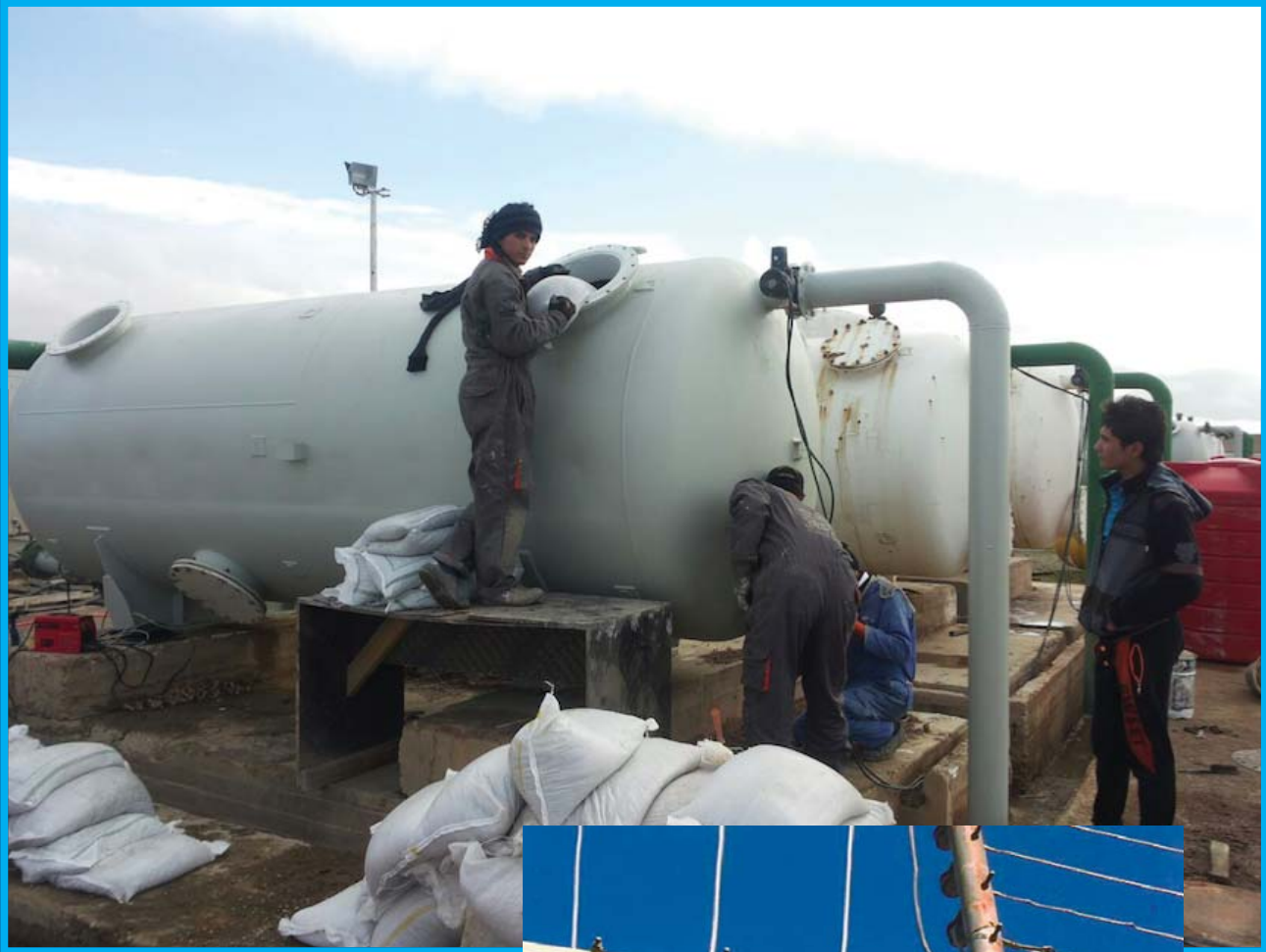
Above: Rehabilitation of the water intake in Tikrit.
