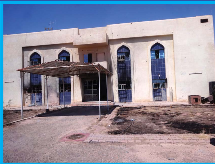
Left: The Qadisiya police station before refurbishments. The interior was completely burned.
