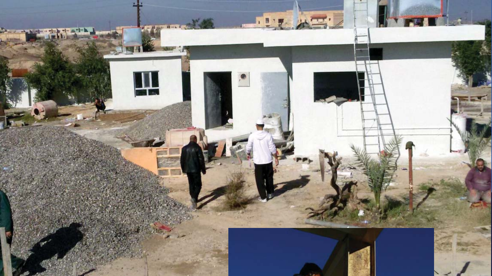
Above: Rehabilitations ongoing at the Tikrit Central Water Station.
