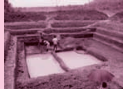
2.5.4 Construction of 5 percent model going on
