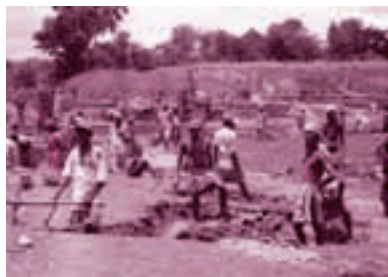
6.4 Work under NREGP going on
